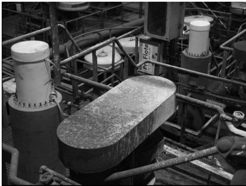
Figure 1 – ProFlote® installation at copper rougher conditioners
